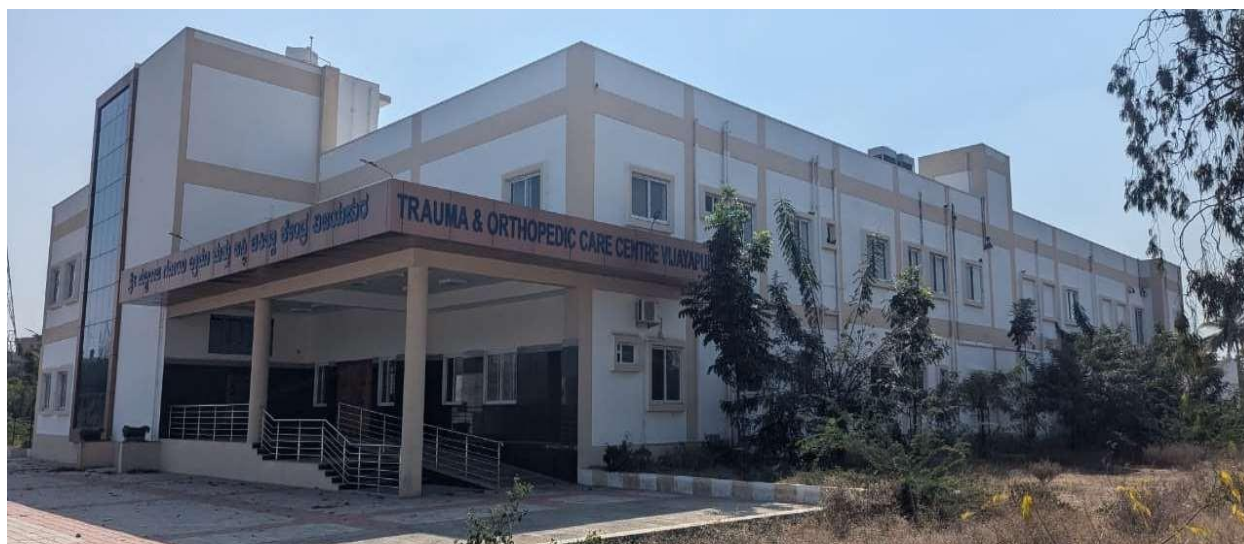
Newly constructed Trauma & Orthopaedic Care Centre
